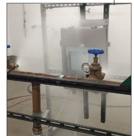
Water Ingress Testing
