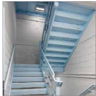
Millenium Round and MOS fixtures in the Brooklyn Battery Garage
