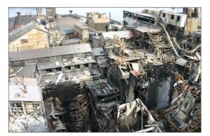
Sugar dust explosion at Imperial Sugar in Port Wentworth, GA. Combustible dust is in Class 2.
