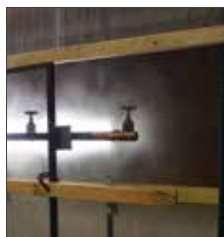
100 PSI Water Test
