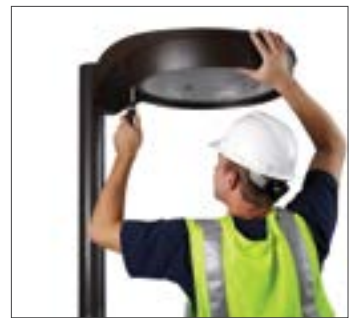
4. Swing the lower hinged portion of the fixture upward. Secure the lower to the upper portion of the housing using the captive screws in the lower housing. Installation is complete.
