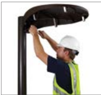
1. Remove the lower portion of the housing. Fasten the upper portion to the pole, using the square pole adapter plate if necessary. Feed the appropriate wiring through the center opening.
