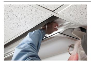
Re-lamp fixture with appropriate lamp wattage type or replacement gear tray.
