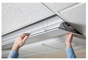
5. To return lens assembly back to closed position, push one long side lens assembly back into the housing, then holding on to the lens repeat on the other side.
