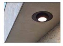
A custom trim ring covers a gap around the luminaire that was left when the larger HID was removed.
