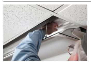
Re-lamp fixture with appropriate lamp wattage type.
