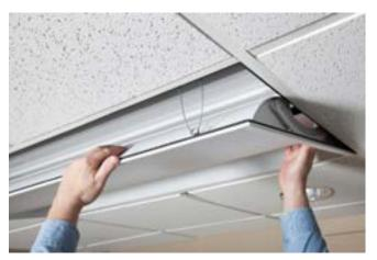
To return lens assembly back to closed position, push one long side lens assembly back into the housing, then holding on to the lens repeat on the other side.
