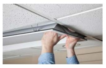
2. Both sides of the lens assembly should be on the down position (as shown) before re-lamping.
