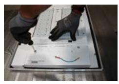
Make all electrical connections from a sealed conduit fitting or bushing to prevent condensation from entering the luminaire.
