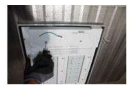
14. LEDs are sensitive and must be protected. Do not place the electrical assembly face down on any surface other than the Top-Base, as intended.
