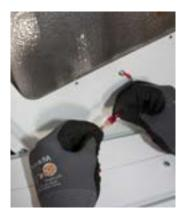
13. Secure wireway cover so that all wires are contained within the compartment.
