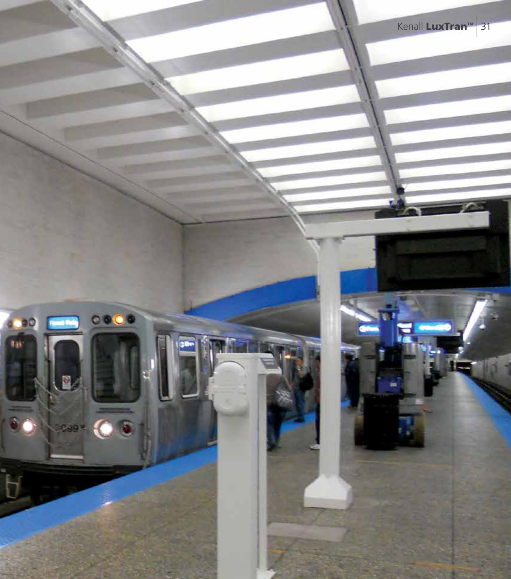
PROJECT: Logan Square Station LOCATION: Chicago, IL PRODUCT SPECIFIED: MLHA12 Series
